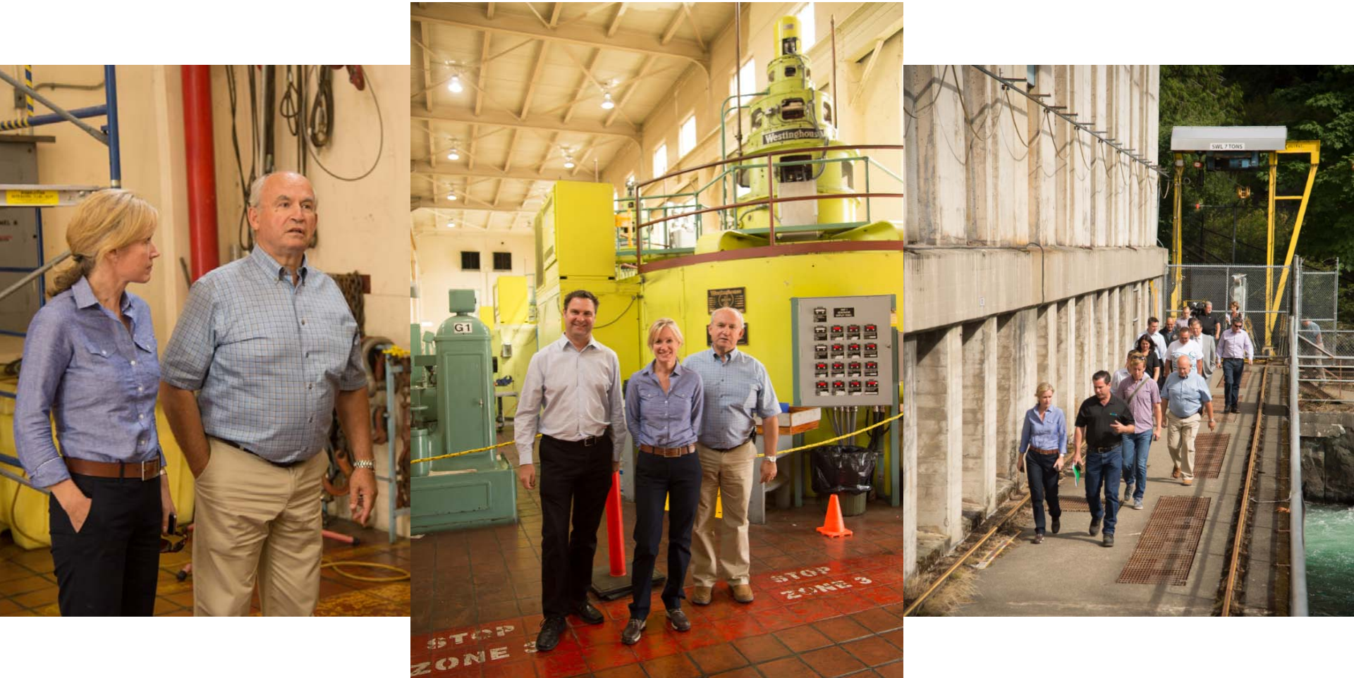
Tour of the John Hart generating station facilities.
