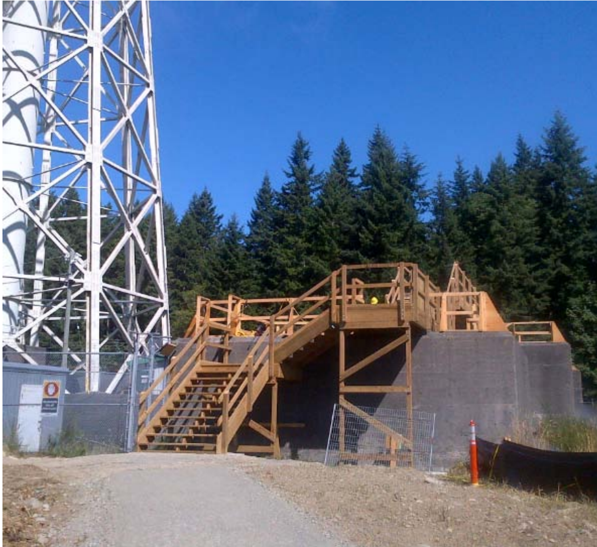
Pedestrian bridge construction.
